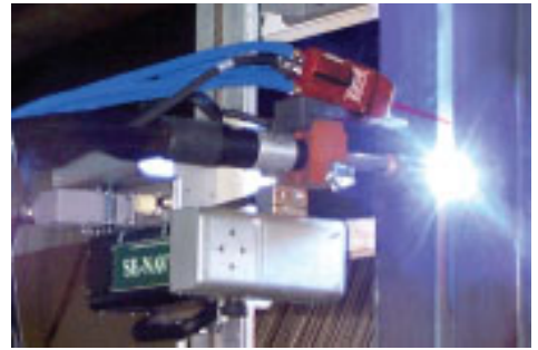
Portable Robot for On-site Ship welding
